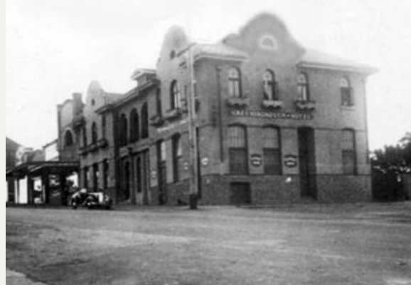
FIGURE 4. Original Greensborough Hotel c1865; 'new' Greensborough Hotel c1913
