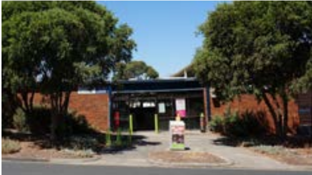
Site photo: View looking east towards entry to arcade
