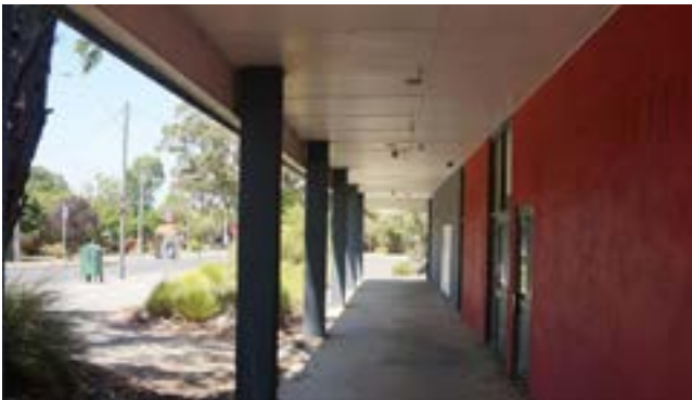
Site photo: View looking along the northern interface of shops
