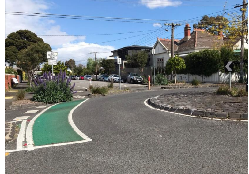
Dwyer St, where only people cycling can exit the roundabout on one of the arms, Clifton Hill VIC
