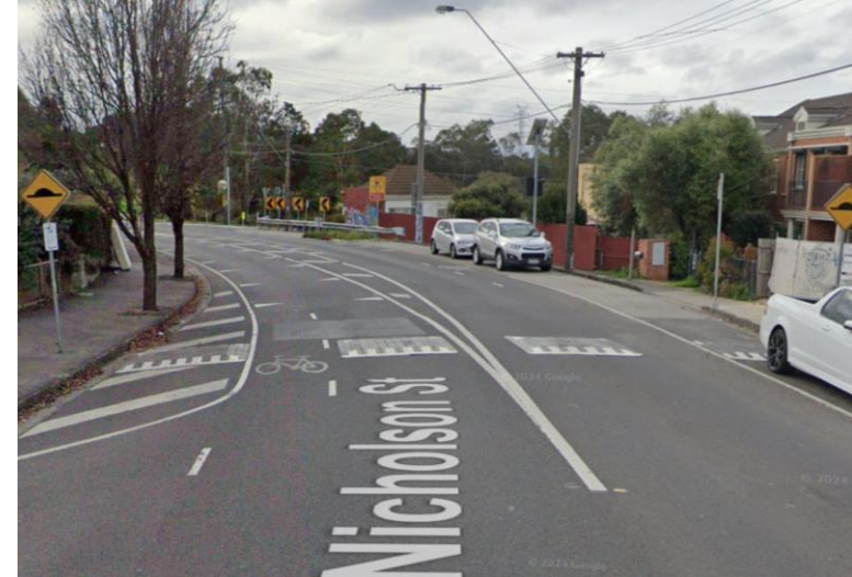
Speed humps on corner approach, Brunswick East, VIC
